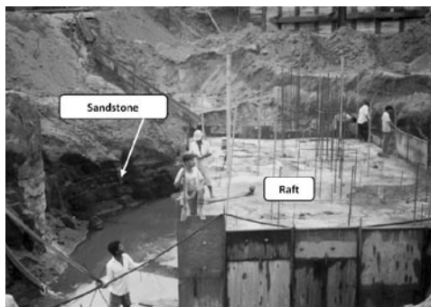
Figure 06: Exposed sandstone upon which raft is founded.
