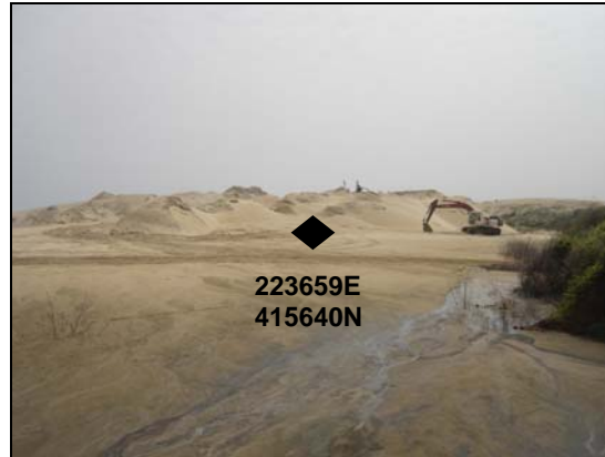
Plate – III: Piled up sand (after refining mineral sand) at Pulmuddai
