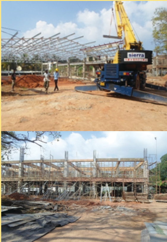
The progress of the 'state-of-the-art' phase IV building of the Faculty of Medical Sciences in January 2015
