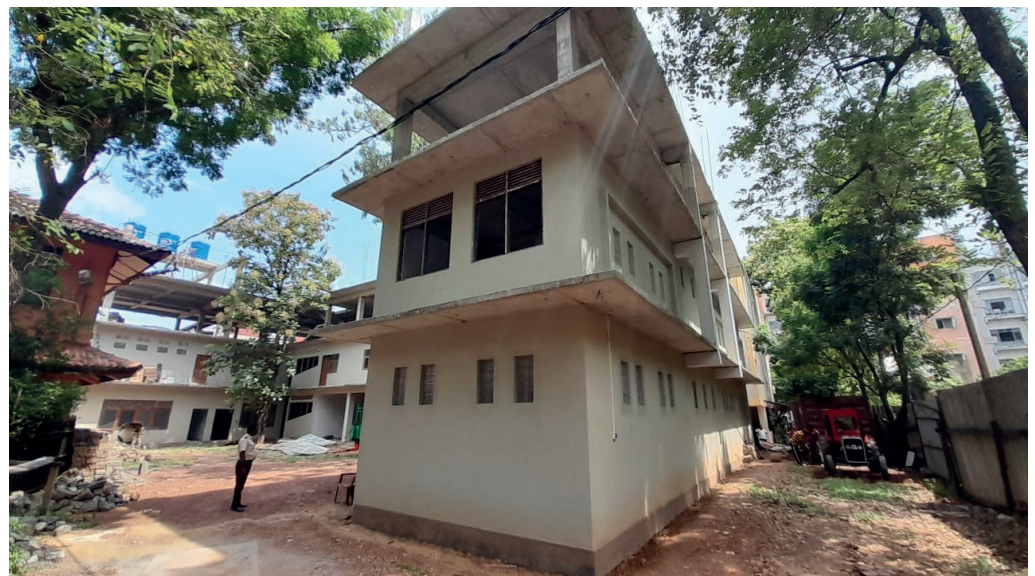
Construction of the New Building for Land Building and Infrastructure Development Division
